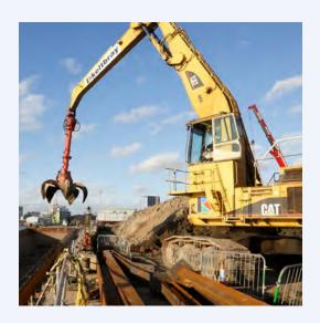
The material was excavated, analysed and then treated depending on the contaminant, which required a high level of performance in terms of treatment capabilities, health and safety performance and operational procedures. In under a year, Keltbray received, treated and recycled 45,000 tonnes of waste soil from the project.
